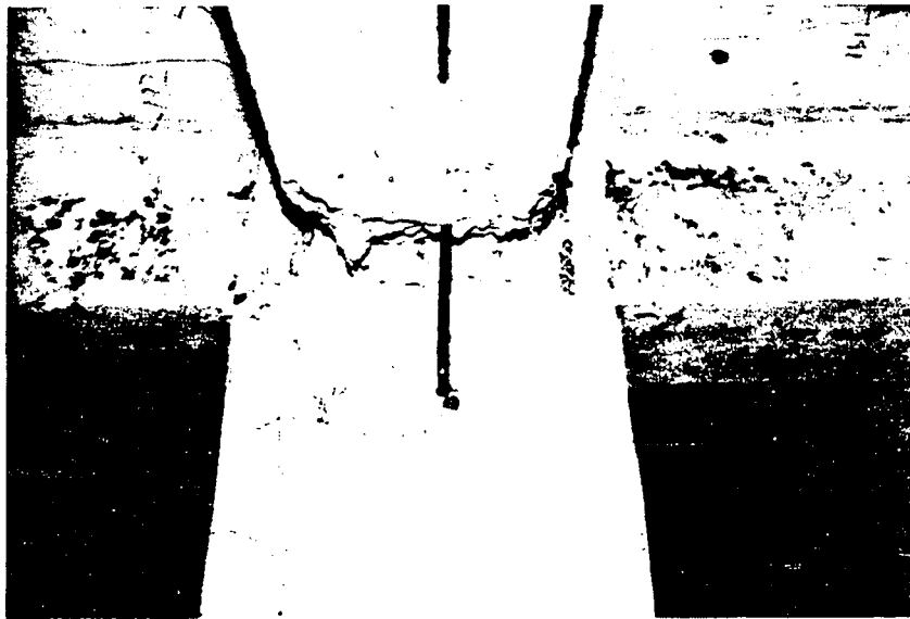
Fig. 3.30 View of joint region at end of test, interior modified
