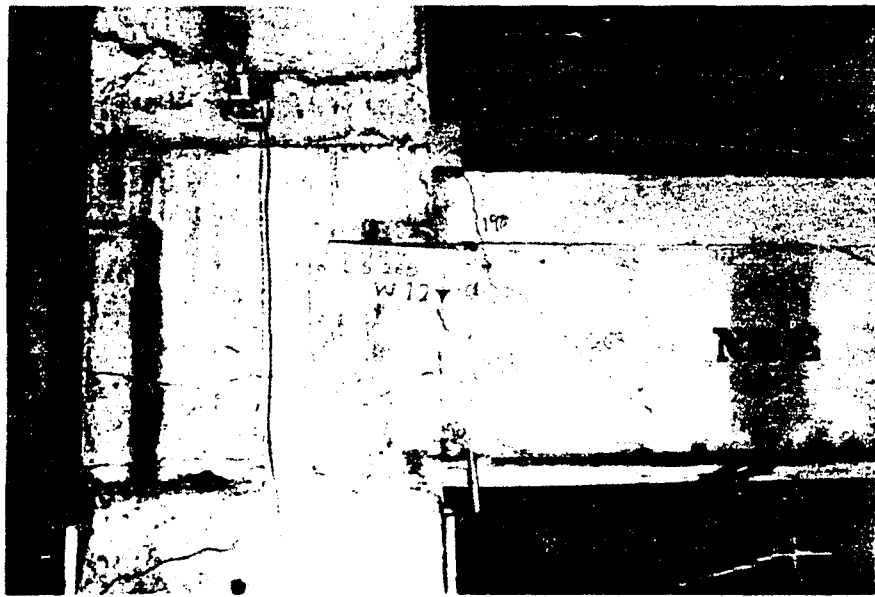
Fig. 3.37 Transverse beam east face at D1.2, exterior modified
